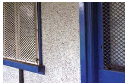
Figure 33 Chrysotile pebble-dash exterior wall coating
