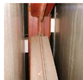
Figure 22 AIB offcuts used as packers around column in CLASP building
