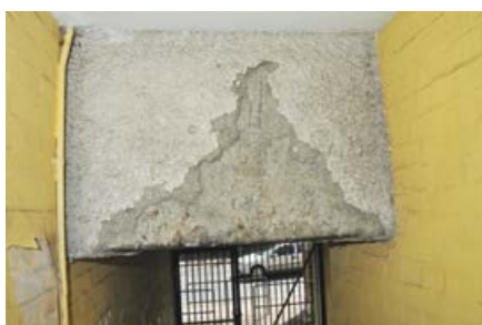
Figure 8 Sprayed coating on building passageway
