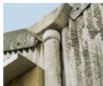
Figure 35 Asbestos cement downpipe
