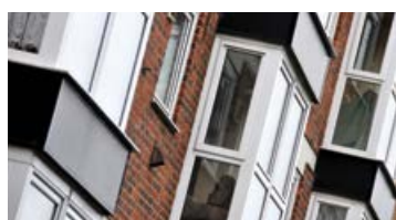
Figure 16 AIB exterior painted panel
